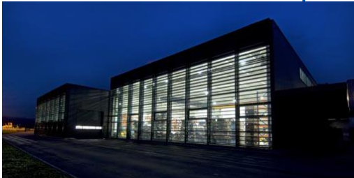
Expansion of production by plant 4
